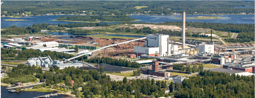
Figure 7 Alholmens Kraft power plant. Source 25
