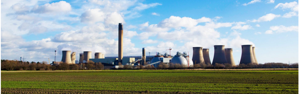
Figure 2 Drax power plant. Source 8
