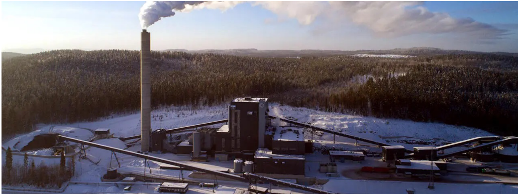
Figure 8 Keljonlahti power plant. Source 30
